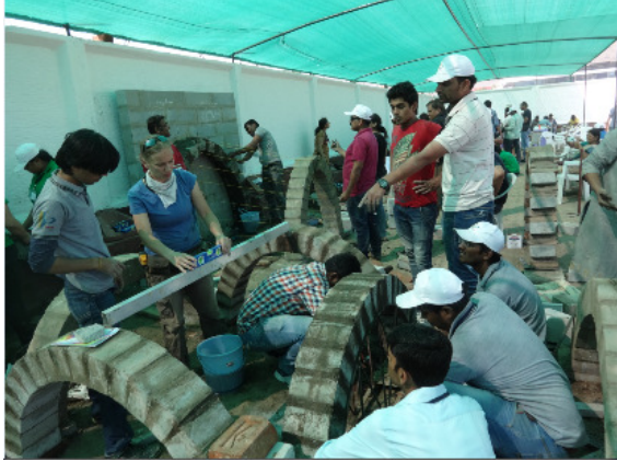
Levelling of pendentive Dome
