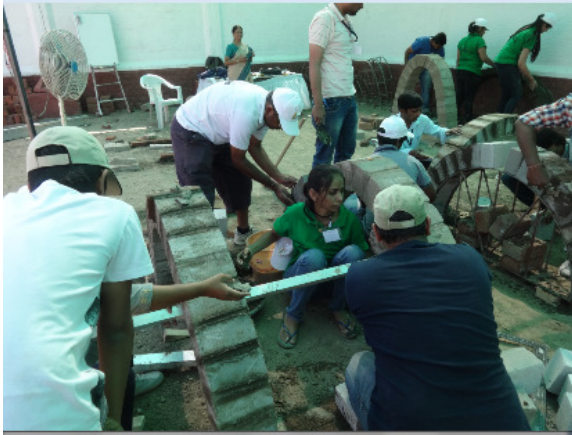
Leveling of semicircular Vault
