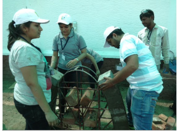
Laying of Bricks
