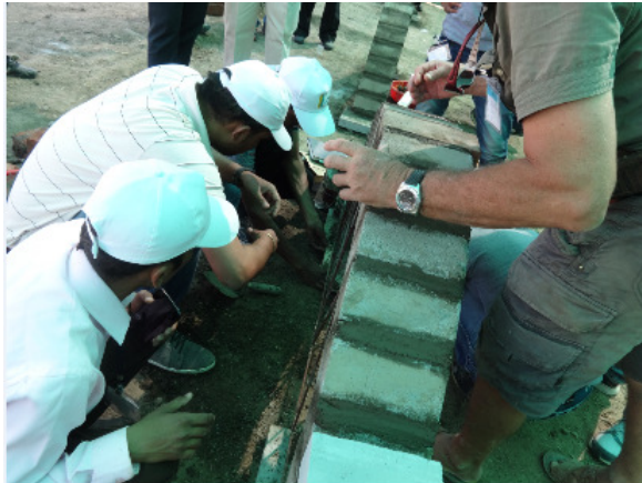
Removal of centering
