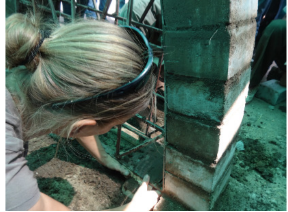
Removal of centering
