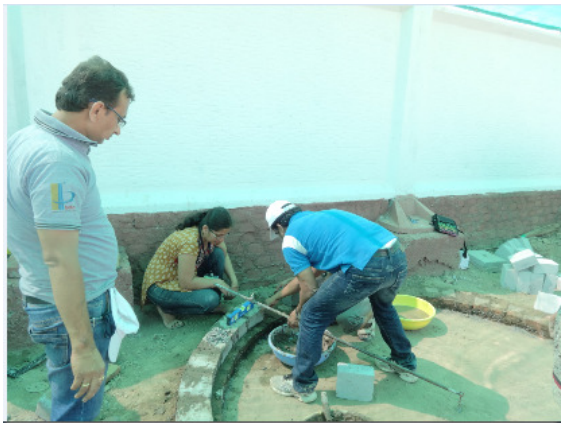
Alignment and leveling of bricks (Igloo)
