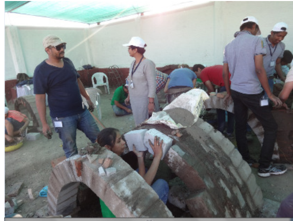
Alignment of bricks (Semicircular vault)
